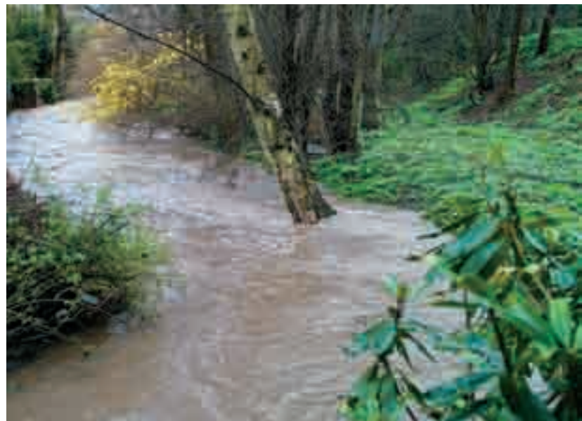
After torrential rain this brook at Trentham became swollen and caused flooding in nearby gardens. This is the type of potential flooding and surface water problem which needs to be identified.
