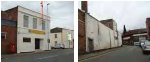
Smaller, less elaborated industrial buildings clearly define streets and spaces and provide a high degree of enclosure
