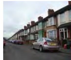
This typology is set back from the edge of pavement to allow small bay windows and front gardens.
