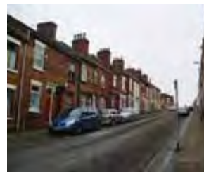
The roof line of this terrace reflects the topography.
