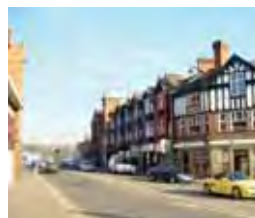
3 Buildings in Burslem are predominately historic in character. This creates a distinct character and opportunity for heritage led regeneration.
