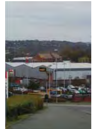
Due to the topography and location of the industrial uses, the roofscape is often very prominent.
