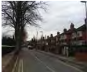
This is an example of a higher quality development, where streets and space are well overlooked and enclosed.
