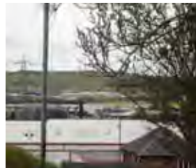
Due to the topography and location of the industrial uses, the roofscape is often very prominent.
