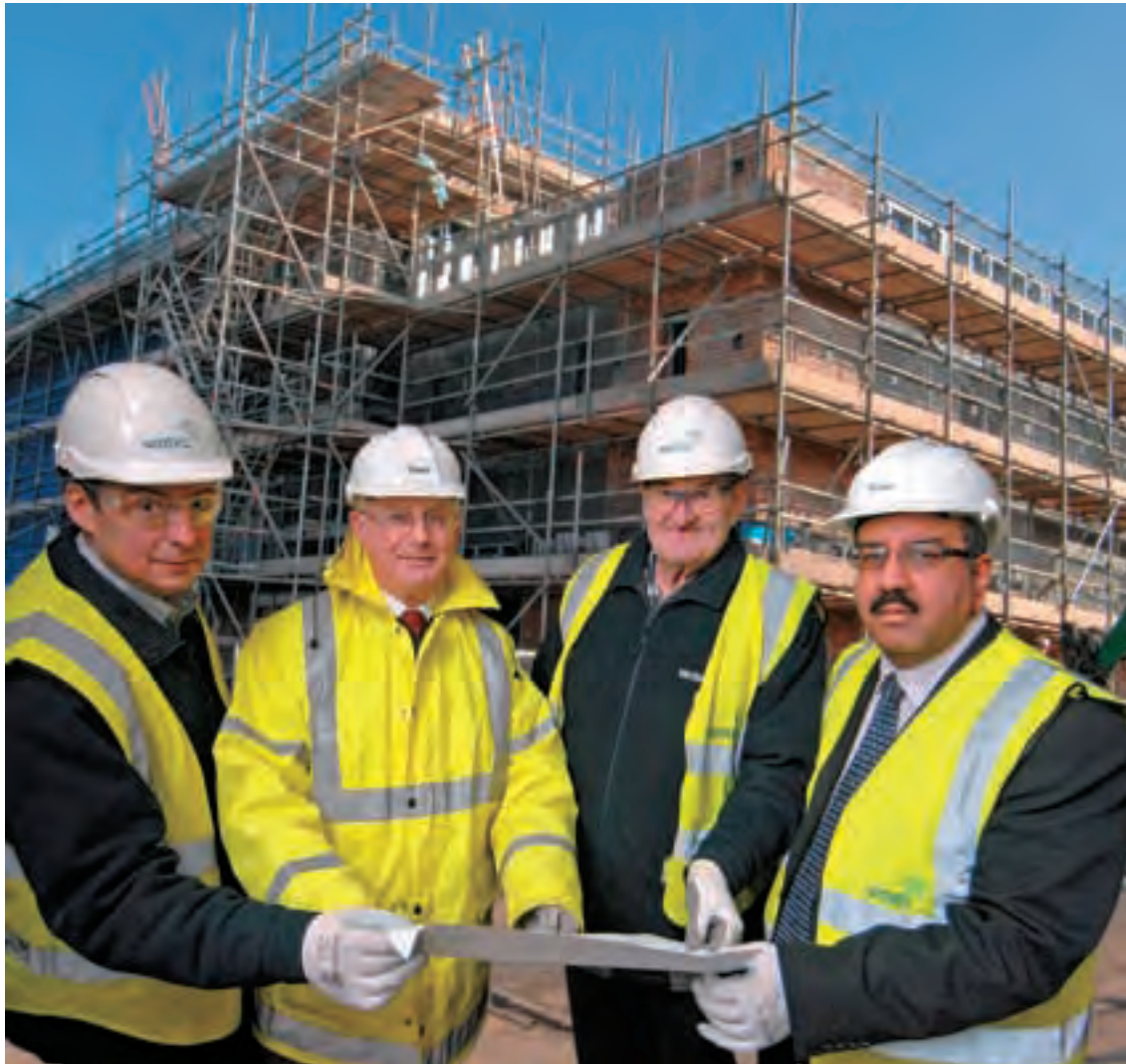
OVERSEEING PROGRESS: city council Leader, Councillor Mohammed Pervez, right, and Patients Group Chairman Bernard Wragg, second right, are given an inspection tour of the Cobridge Health Centre construction site by Steve Warden, Project Manager for builders Wates, left, and Campbell Boyle, Chairman of Prima.
