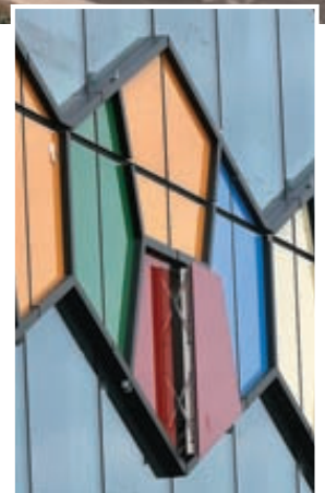
Smithfield Two with its distinctive coloured honeycomb-shaped glazing. Below right, sections of the honeycomb glass open outwards to let in air.
