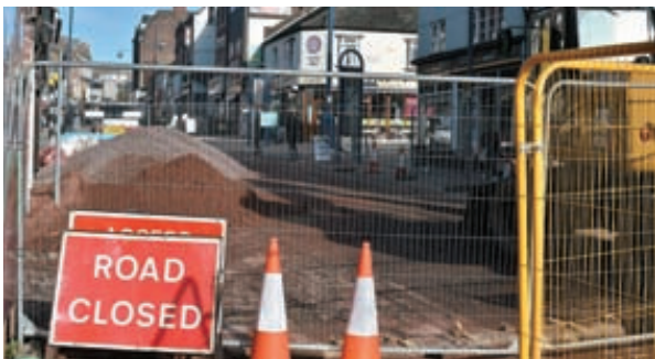
Landscaping work is underway in Piccadilly.
